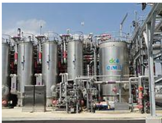
Figure 33: The thermal hydrolysis system at the Blue Plains treatment plant in Washington, D.C.
